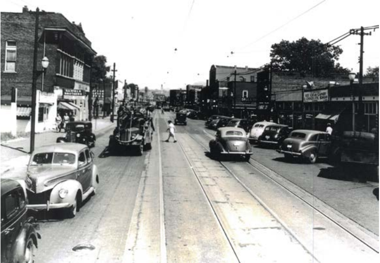
View of Kansas Avenue from 7 th Street, Armourdale Neighborhood
